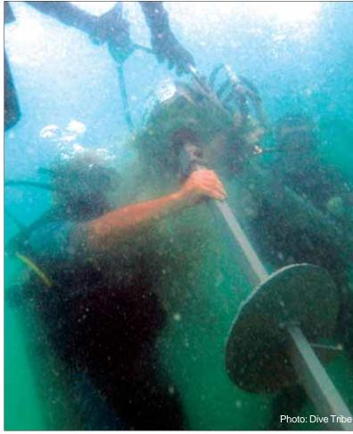
Go Eco Phuket in the process of installing the new style mooring screws.
