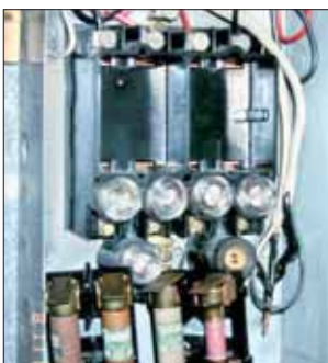
Bypassing the fuse can start fires. Photo: Inspectapedia
