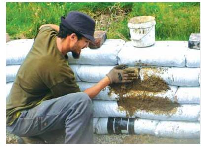
The earth bag construction method requires minimal manufactured materials and minimal skilled labor. Photo: KaneJamison.com
