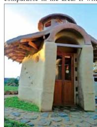
A building constructed from rammed earth. Photo: Bomun
