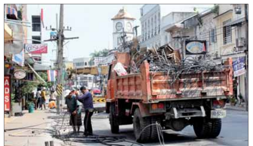
Having buried the power supply cables PEA workers will begin to remove the utility poles from along Phuket Road. Photo: Kritsada Mueanhawong
