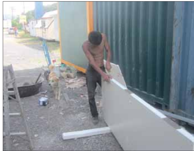
A laborer cuts a piece of insulated panel, which allows for a quicker 'speed of erection' compared to conventional methods.
