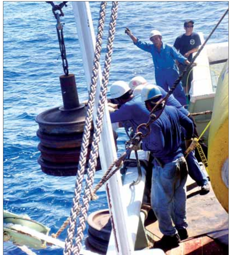
ANCHOR AWEIGH: Crewmen lower a massive anchor that was sunk to tether the buoy to the seabed 3,000 meters below. Photo: PMBC
