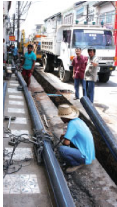
GOING UNDERGROUND: Workers lay underground electricity cables along Talang Road in Old Phuket Town.
