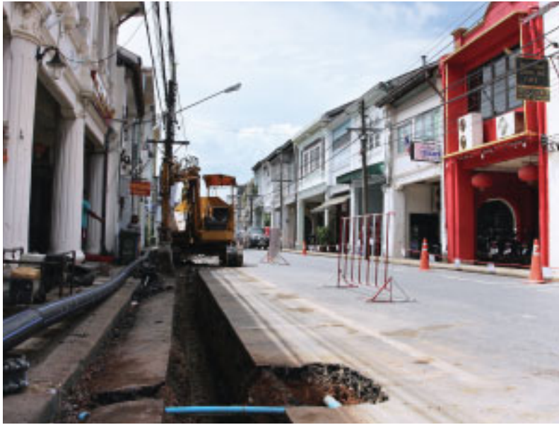
MEN AT WORK: As of June 3, workmen had begun digging a trench for the new HDPE water pipe. A separate trench is to be dug for the power cables on the other side of the road.
