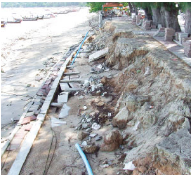
TIME AND TIDE: A view of the damaged seawall built just five years ago.
