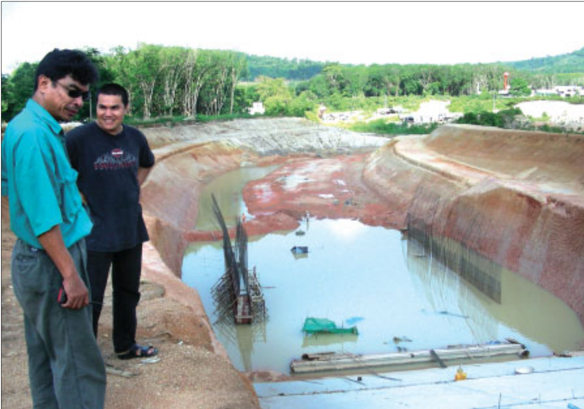
This large concrete spillway will allow excess water to run off safely into Klong Bang Neaw Dum during the rainy season.
