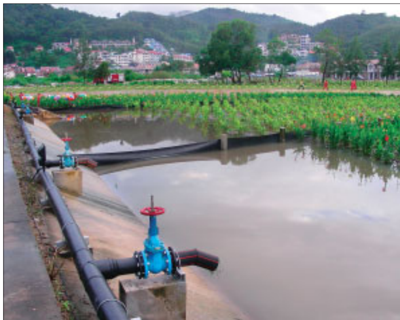
SEAWEED DIET: At the 13-million-baht natural wastewater treatment plant, Canna plants will absorb much of the organic waste that used to flow into Patong Bay, feeding the seaweed there.
