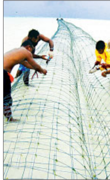
Preparing a Biorock mesh.
