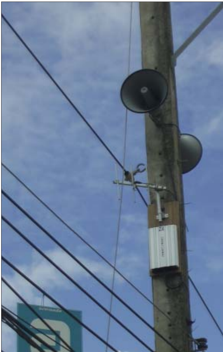
Patong Municipality's warning system, consisting of loudspeakers attached to power poles, was the first to be wired up, but it is not linked to the National Disaster Warning Center in Nonthaburi.
